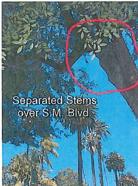
Dangerous Elm over S.M. Blvd.
