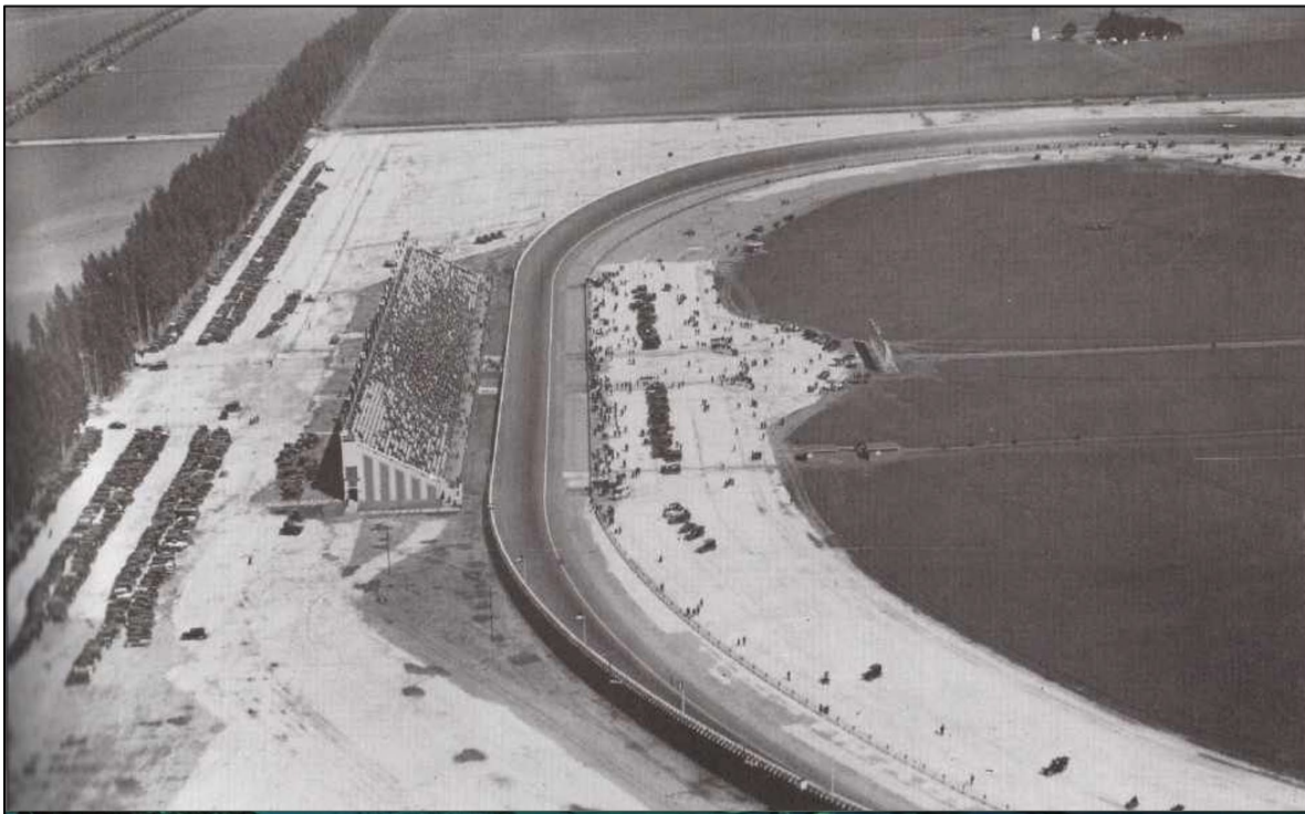
Aerial view of Grandstand "B," race track, parking area, and main entry drive, looking east
